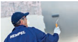
Apply Hempel's Underwater Primer onto prepared surface
