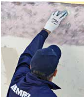
Fill along boottop
