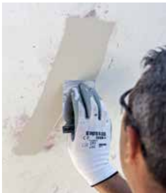
Fairing any defects
